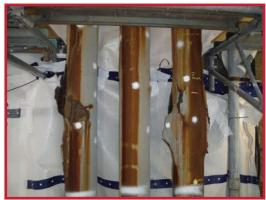
**BEFORE:** This 69 kV electrical feeder system was coated with lead paint and coal tar mastic, contained multiple barrel repairs and was leaking nitrogen.
