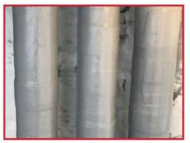
**AFTER:** Carbon Fiber Engineered Solutions installed a custom designed solution while the system remained in service. The new system reduced nitrogen replacement costs by \$250,000 over the first year and extended the life of their existing feeder system by 30 years.
